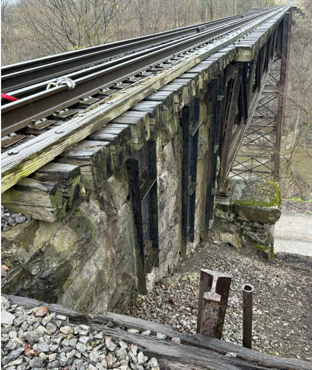
Bridge 15.85 over Eden Eighteen- Mile Creek, Town of Eden
